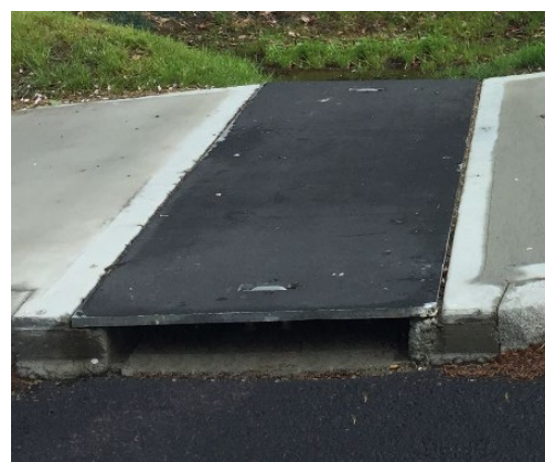
Installation of depressed concrete pad in front of inlet curb opening to create a low point that helps convey gutter flow into the bioswale (left photo). Curb cut opening to direct road runoff beneath the adjacent sidewalk into a stormwater BMP (right photo).
