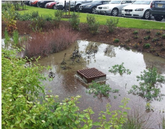
Bioretention basin at the edge of a parking lot.
