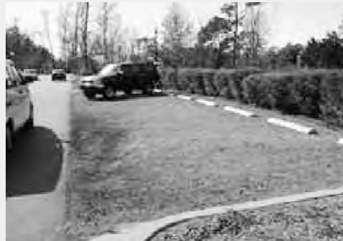
Parking Lot with Porous Surface
